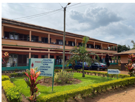
Figure 1 District Hospital of Dschang, Cameroon.
